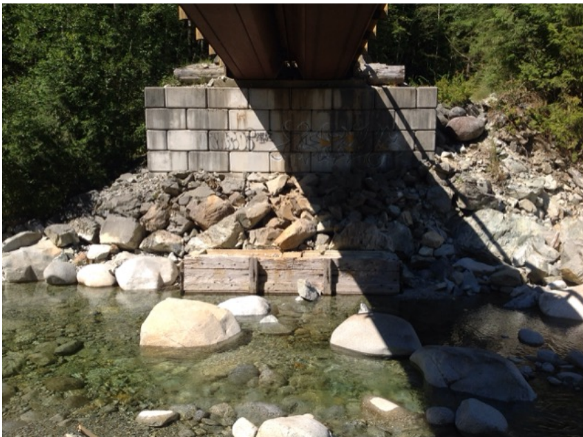
Right Bank Abutment when facing downstream
