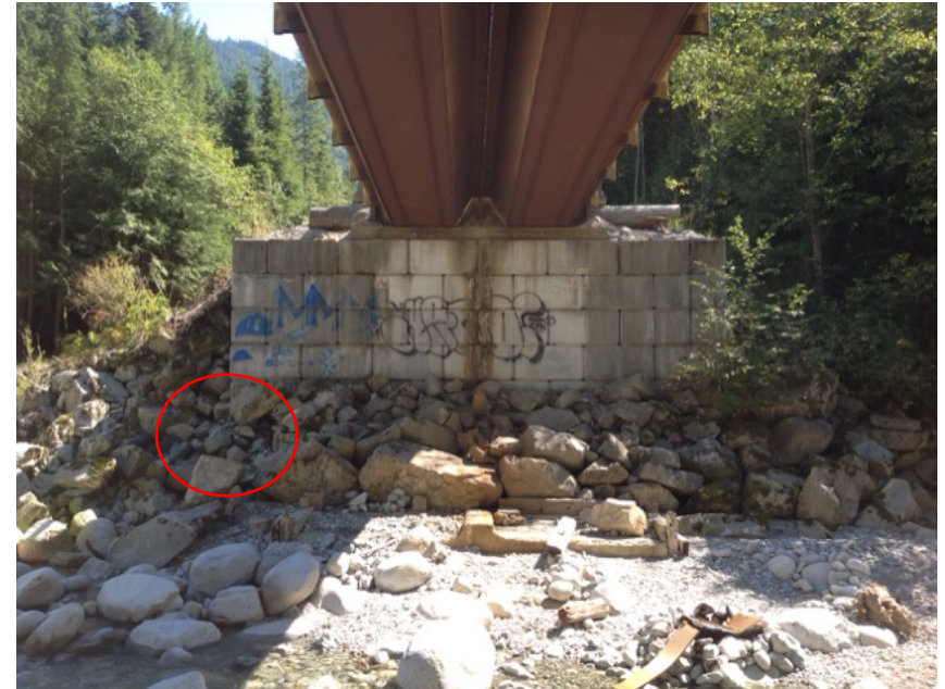
Left Bank Abutment when facing downstream
