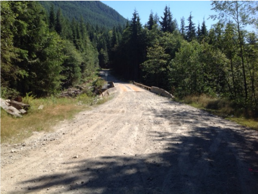
Approach from Right Bank when facing downstream
